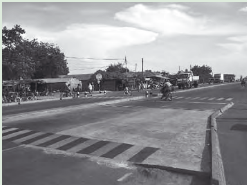
The two raised areas are staggered on each side of the central island to slow vehicles down before the zebra crossings.
